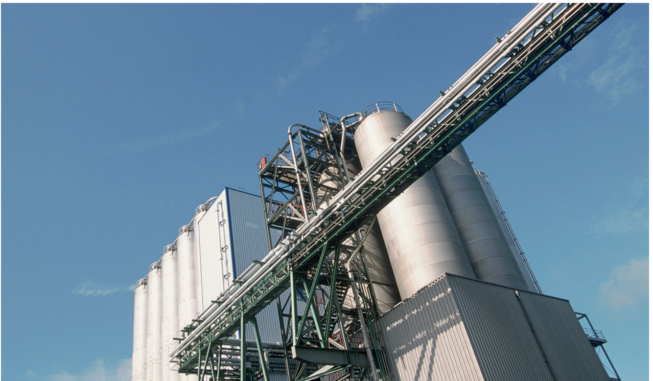
A conveying line from Zeppelin: conveying bulk materials with water represents a product-friendly alternative © Zeppelin
